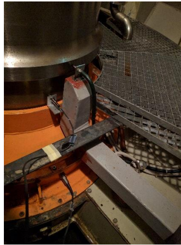
Proximity probes installed on the turbine bearing. Next to the MCM system probes. Accelerometer seen as well.
