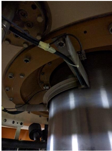
Proximity probes installed below the generator bearing. They're positioned next to the MCM system probes.
